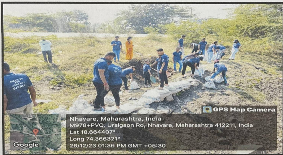
Construction of dam by NSS Volunteers.
