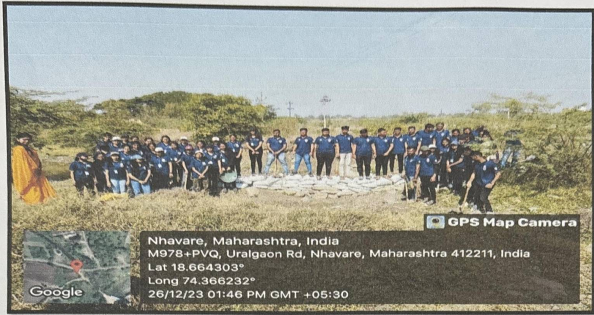
Construction of Bandhara for conserving of water in rainy season.
